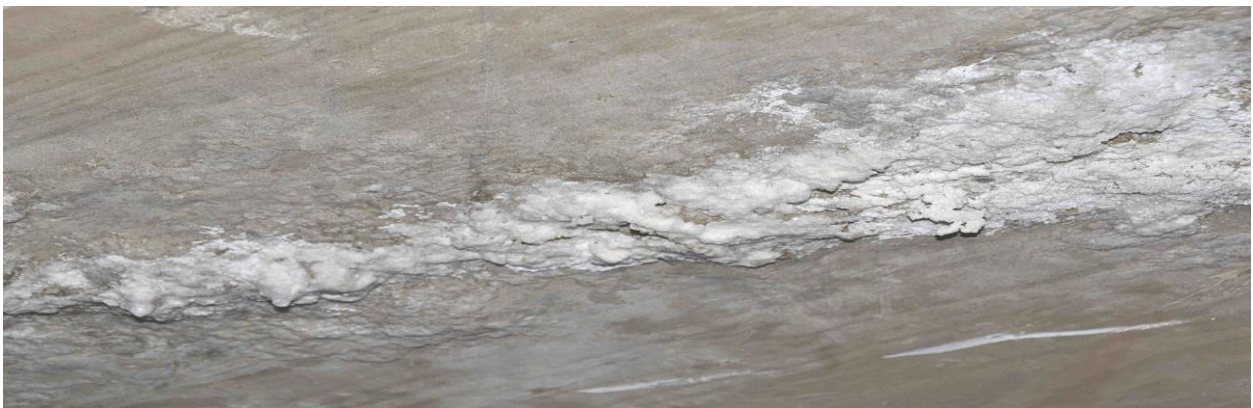
Fig 2 : Example of secondary efflorescence in parking garage exposed to diluted road salt from vehicles entering the garage during winter.
